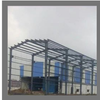
Pre Engineered Building Structure System
