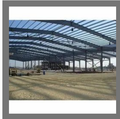
Pre Engineered Building Structure
