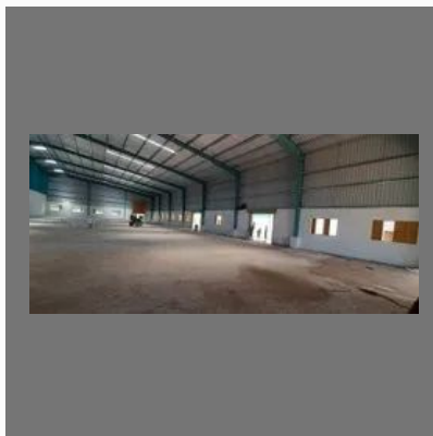
Badminton Court Roofing Shed
