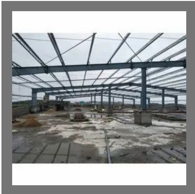
Pre Engineered Building Structure
