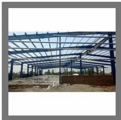
Pre Engineered Mild Steel Building Structure
