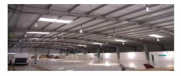
Made of translucent GRI to match Re Group rib and wall panels, with an estimated light transmitting capacity of 60%
